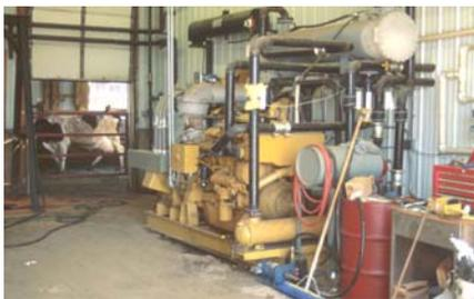
*A generator on a diesel motor converted to run on methane from the digester provides electricity for the Haubenschild farm operations, Princeton, MN.*
